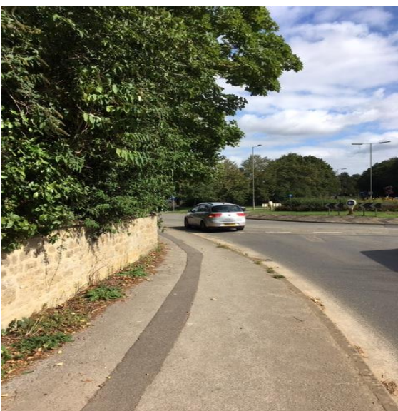
Driver's view of crossing point is obstructed by foliage and wall.
